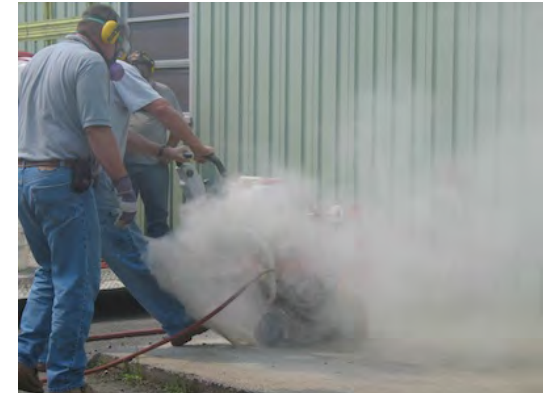
Without water control
