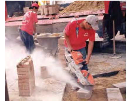
Without water control
