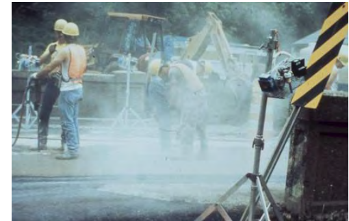
Without water control
