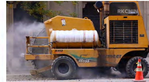
Without water control
