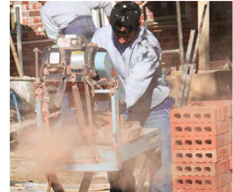
Without water control
