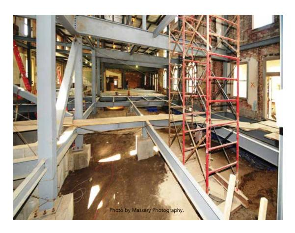
To erect the steel inside Becht Hall, some 200 boles were cut in the roof to allow steel to be lifted into the building. For all the planning and preparation, there was little that could be done to create efficiency.
