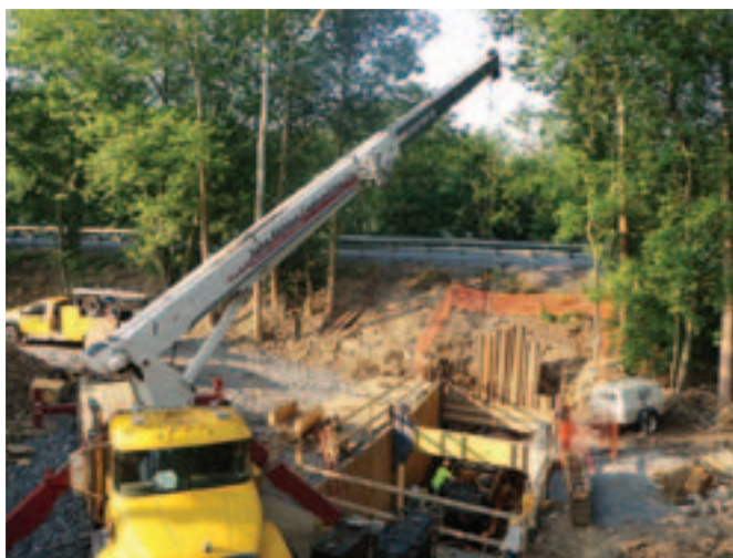
A new 60" effluent pipe was bored under Business Route 22 from the plant to the Juniata River.
