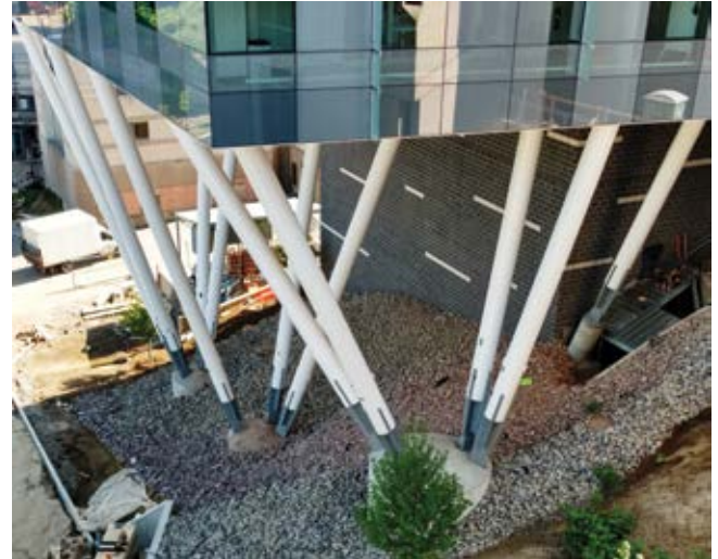
A critical design decision was to elevate the first level of Scott Hall on steel columns three stories above the road at Panther Hollow.
