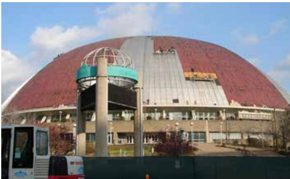
Bristol Environmental performed the removal of the aluminum cladding from the former Civic Arena's roof.
