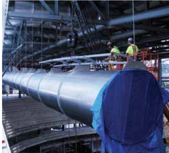
McKamish Inc. installed the bull duct at PPG Paints Arena 150 feet above the ice before the roof of the arena was completed.
