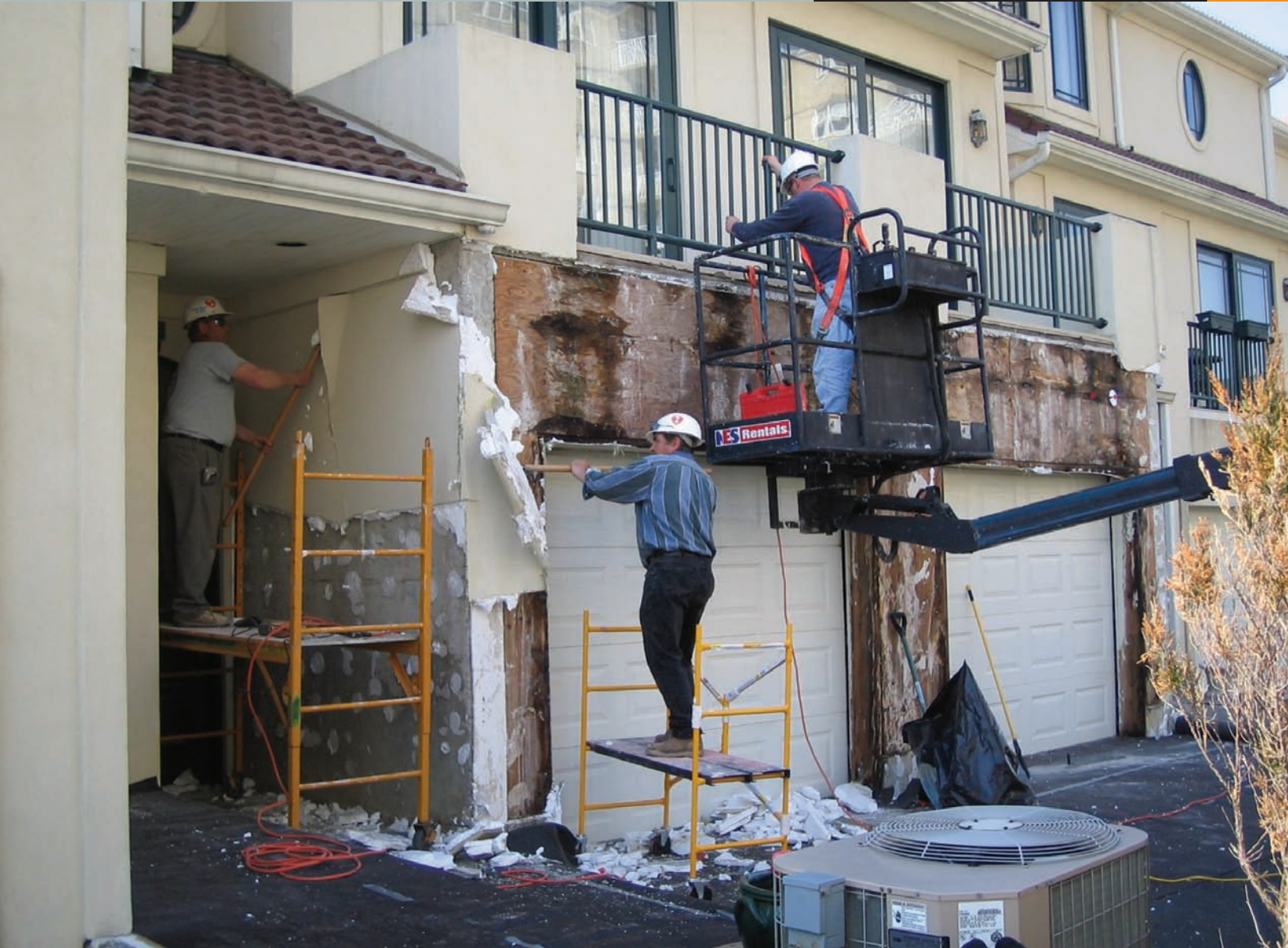
Robson expert examines water infiltration damage behind failed EIFS exterior.
