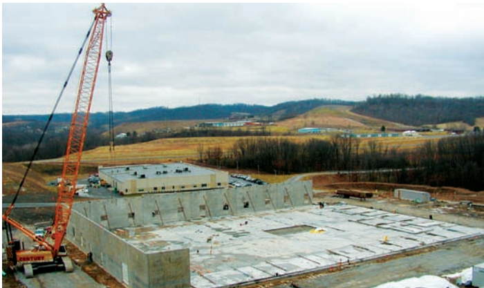
Site cast panels for the exterior of the second building at EverGreene Technology Center are lifted into place.
