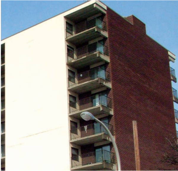
Removing EIFS and railing systems from the 1980's allowed for an exterior with more architectural interest.
