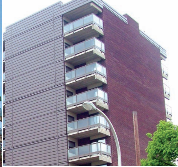
Removing EIFS and railing systems from the 1980's allowed for an exterior with more architectural interest.
