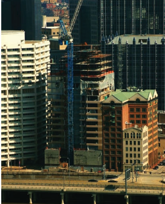
Exterior cladding goes onto the skeleton of the 18-story 151 First Side Condo
