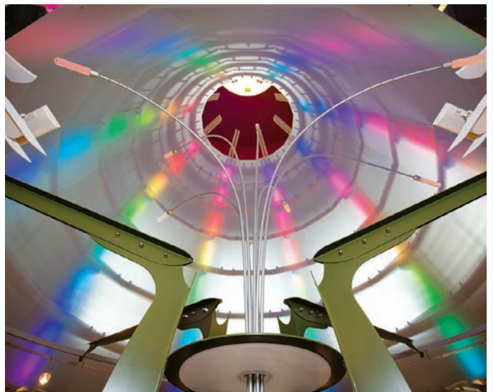
Laminate columns from Seech Industries are covered with translucent ‘eco-resin’ from 3form® (photo by Ed Massery).
