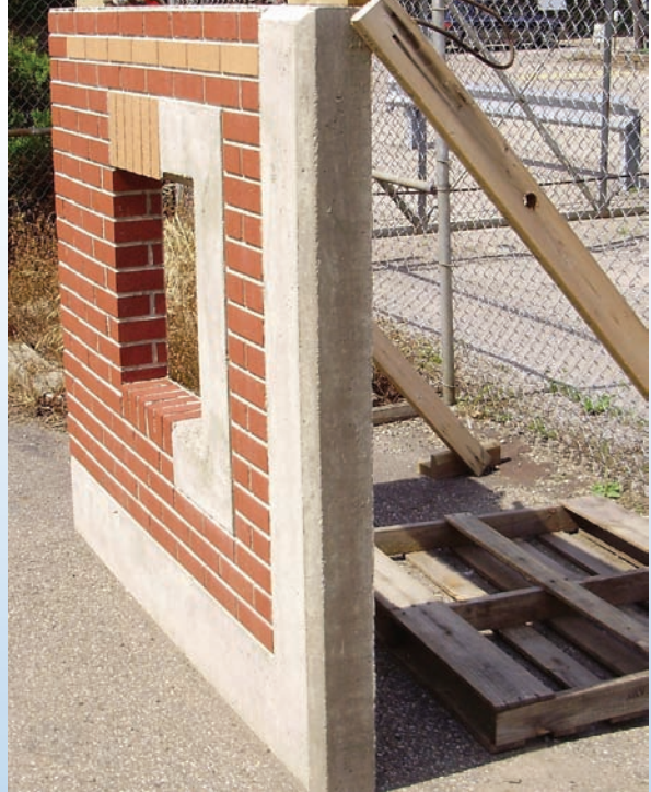
Architectural elements and traditional finishes like brick can be embedded in the panels during the horizontal pour (mockup photo courtesy of Burchick Construction).
