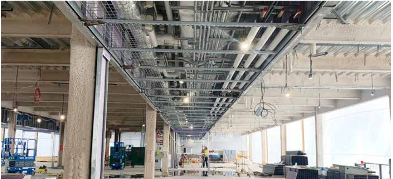
Site conditions varied dramatically between the floors that had the prefabricated racks and the lower levels that were constructed conventionally. Photo by W. G. Tomko Inc.
