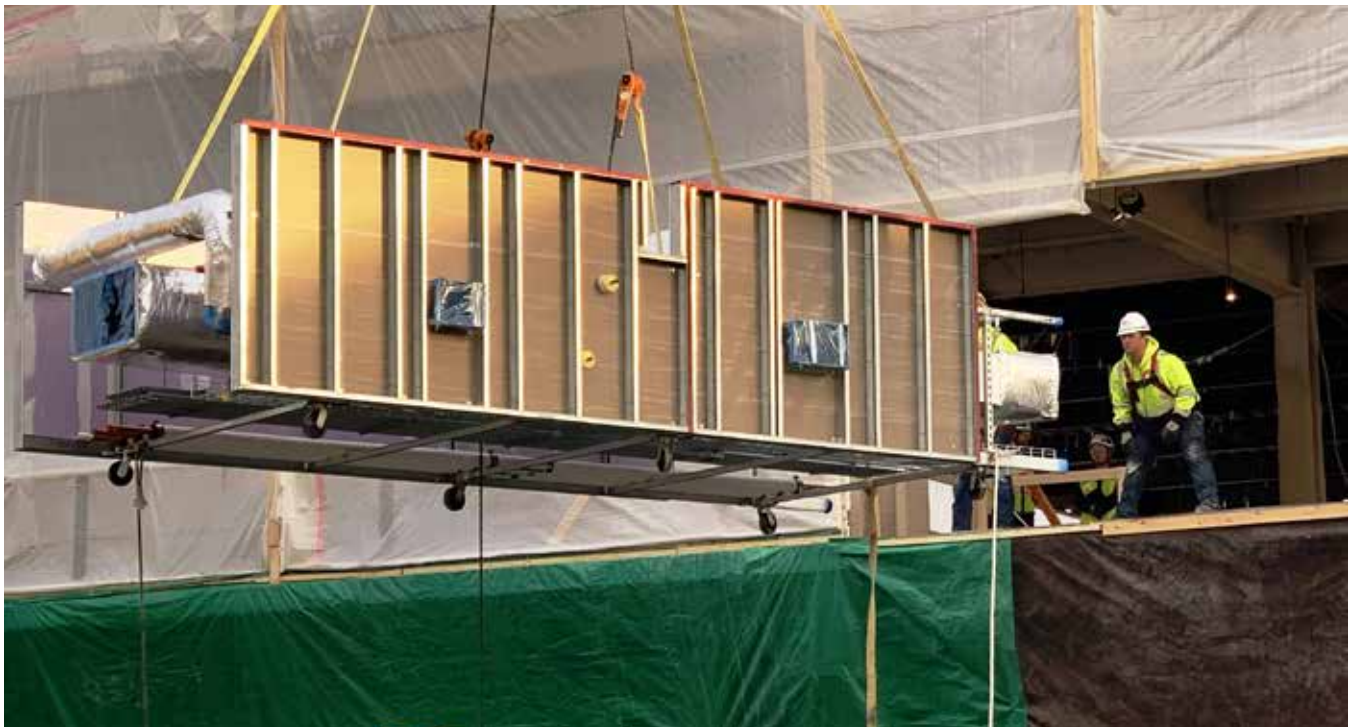
Fully fabricated rack sections were lifted onto the hospital floor for installation through temporary "docks" in the building's exterior walls. Photo by W. G. Tomko Inc.
