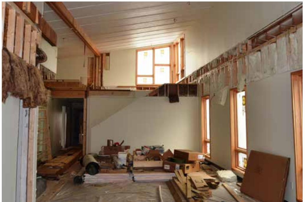
Each module was delivered to the site with finished interior walls, ceilings, flooring, and trim. Photo by Jendoco Construction.
