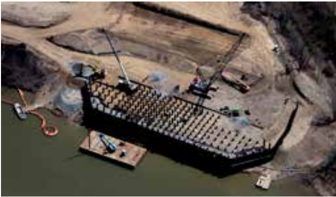
New marinas were built at the north and south ends of the facility to allow prefabricated sections of the plant and other construction components to be shipped up the Ohio, and to ship polyethylene out once the plant is operational.
