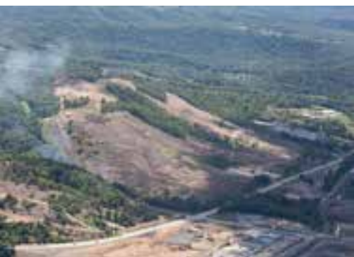
Trumbull moved nearly seven million cubic yards of earth to make a wooded hillside into a flat plant site.
