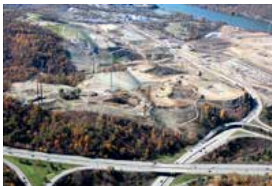
Trumbull moved nearly seven million cubic yards of earth to make a wooded hillside into a flat plant site.
