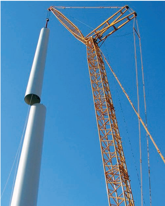
Cranes lift a section of the 80-meter turbine tower (Photo Courtesy Walbridge East).
